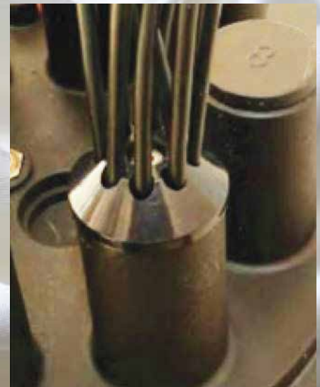
Drop cable sealing
